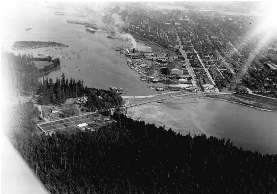
Fig 13. An aerial view of the causeway under construction showing Lost Lagoon separated from the rest of Coal Harbour. “Showing Entrance to Stanley Park looking East,” May 27, 1919. Stuart Thomson fonds, AM1535-S1-: CVA 1123-6, City of Vancouver Archives.
